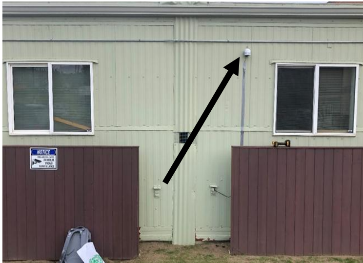
Figure 4. Exterior Sensor Setup @ Facility 1
