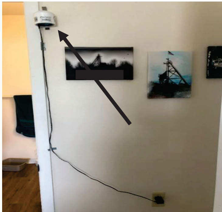
Figure 5. PurpleAir Setup @ Facility 2
