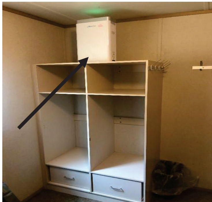
Figure 3. PAC Setup @ Facility 1
