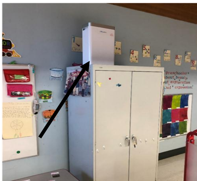
Figure 9. PAC Setup @ Facility 3
