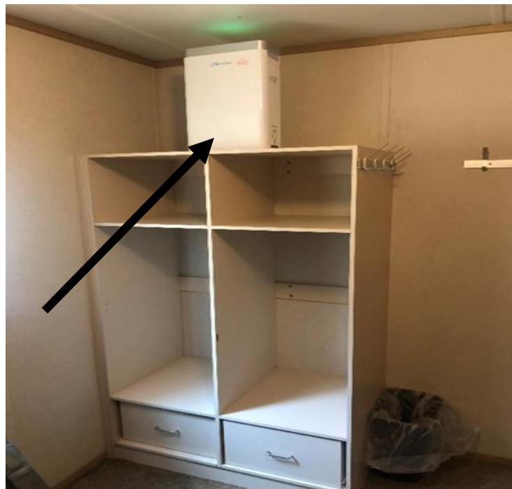
Figure 3. PAC Setup @ Facility 1
