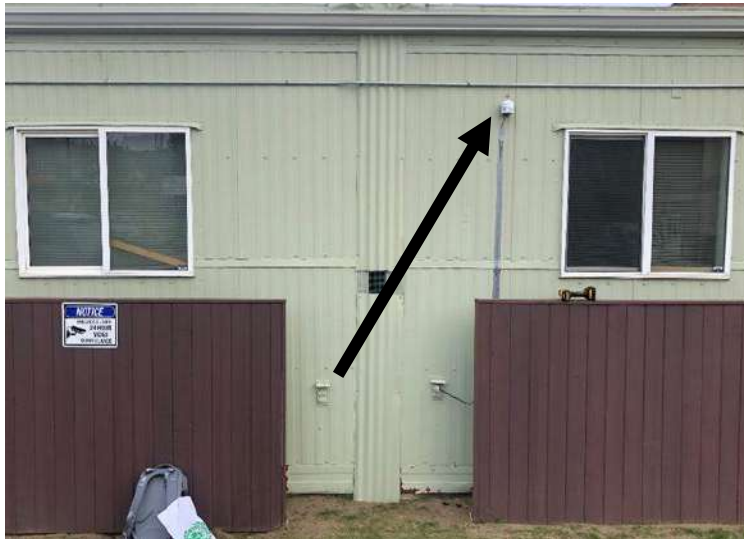
Figure 4. Exterior Sensor Setup @ Facility 1
