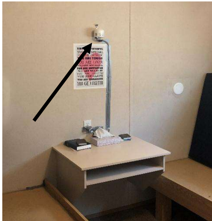
Figure 2. PurpleAir Setup @ Facility 1
